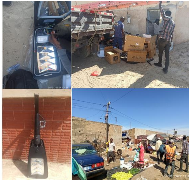
Figure 25 | A Few Installation Steps in Diamaguène, (© IfaS)
