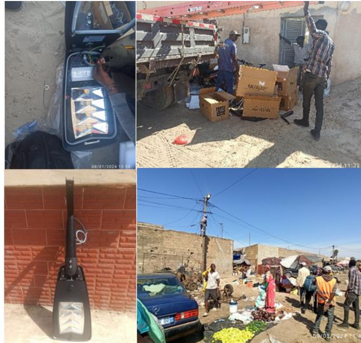
Figure 50 | A Few Installation Steps in Diamaguène
