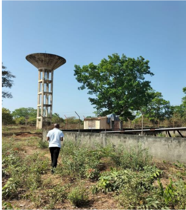
Figure 6 | Presently Available Water Tower, (© IfaS)
